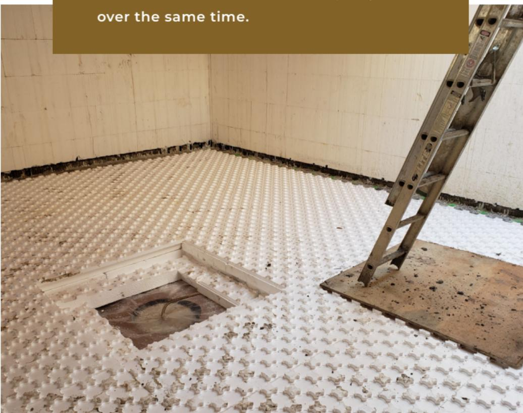
Insulation under basement slab keeps it from feeling like a cold basement floor.
